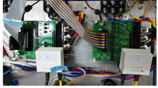
Fig. 10. Two converters connected to the test machine.
