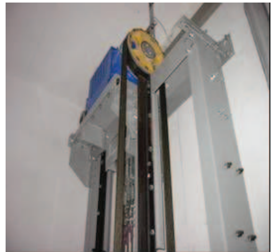
Fig.6. Photo of recent lift the feature of which is machine room less.
